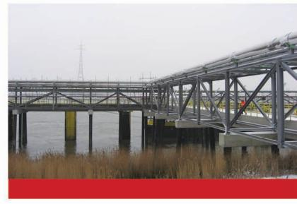
The solution for these requirements was a double layer pipe system of the product series Type FIRESAFE-T60, equipped with fire protection foam insulation and a spiraled inside fold jacket fulfilling all requirements.
