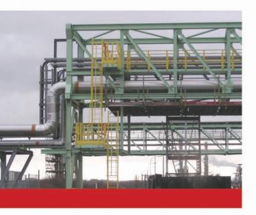
The pipeline crosses over public land. This meant high standards for environmental protection and fire prevention had to be met. The pre-insulated pipe had to have the capability to withstand fire for over 60 minutes. Liquid ethylene operates at -105°C. This low temperature means a large difference to the ambient air temperature. Therefore the pre-insulated pipe design had to guarantee an absolute diffusion resistance.
