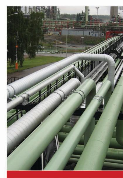
Heating cable runs of between 800 and 1000 m were realised without any cable joint at this refinery in Porvoo.
