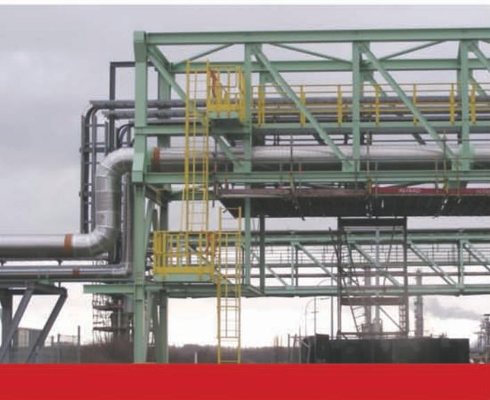
The pipeline crosses over public land. This meant high standards for environmental protection and fire prevention had to be met. The pre-insulated pipe had to have the capability to withstand fire for over 60 minutes. Liquid ethylene operates at  $-105^{\circ}\text{C}$ . This low temperature means a large difference to the ambient air temperature. Therefore the pre-insulated pipe design had to guarantee an absolute diffusion resistance.
